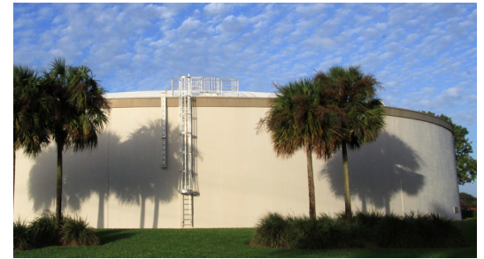
Water Storage Tank at Water Treatment Plant 3
